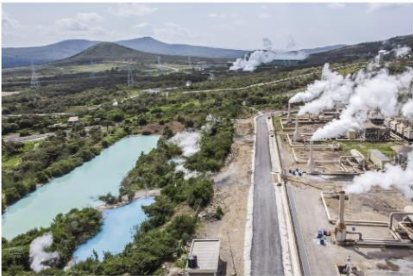
Steam rises from the chimneys of a wellhead plant at the Olkaria Geothermal Complex, operated by Kenya Electricity Generating Company Plc (Kengen), in Hells Gate National Park in Naivasha, Kenya. Photographer: Patrick Meinhardt/Bloomberg
