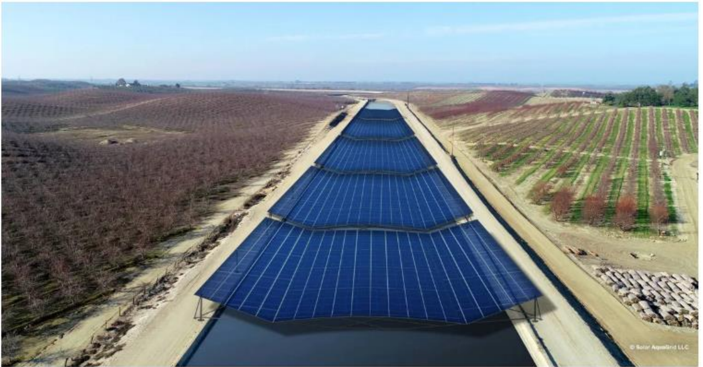
A rendering of a solar-array prototype spanning a canal in Central California (Solar AquaGrid)
