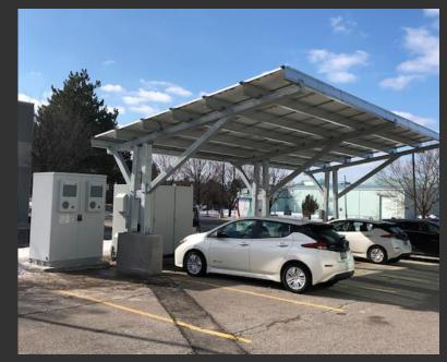
Commercial building in Markham, Ontario Charger: Coritech VGI-30 (30 kW) DERs: 100 kWh/30 kW battery, 6 kW solar 2 Vehicles: 2018/2019 Nissan LEAF
