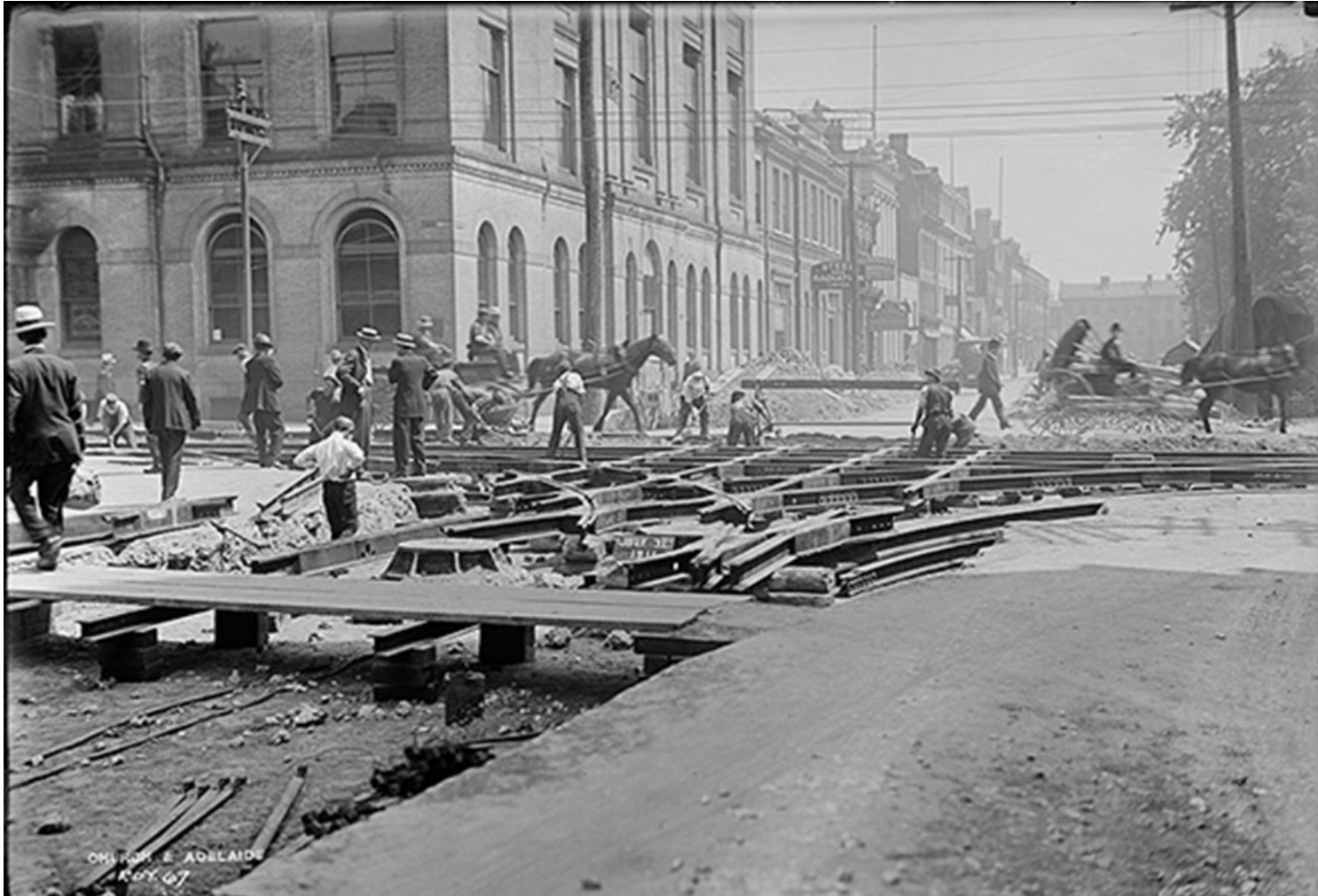
Laying streetcar tracks at Church and Adelaide, Toronto, (Image in public domain, Toronto archives Sens 372, s0372_ss058_it0067.)
