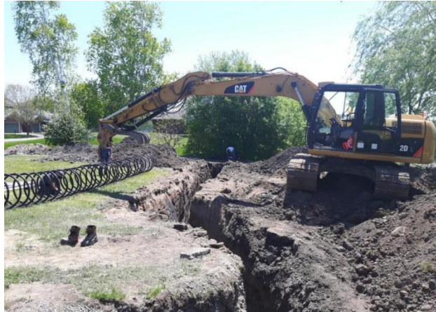
Figure 28: Image showing lowering the ground loop into the trench
